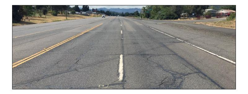
**Pavement:** The four-mile area of Oregon 42 between Lookingglass Creek and Grant Smith Road was last paved in 2006. The pavement shows extensive surface wear and cracking. Turns lanes are heavily rutted.
